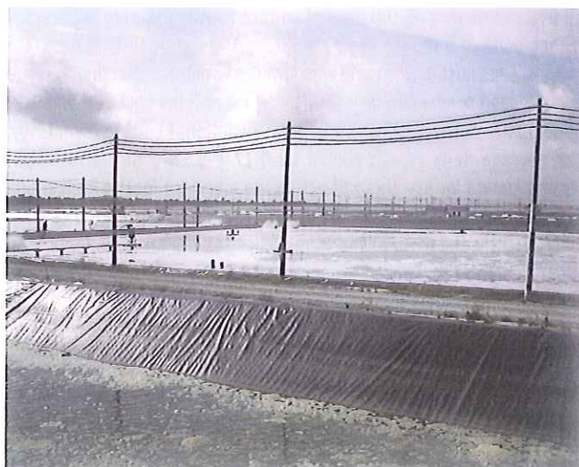
Overview of ponds and supply canal in phase 1
